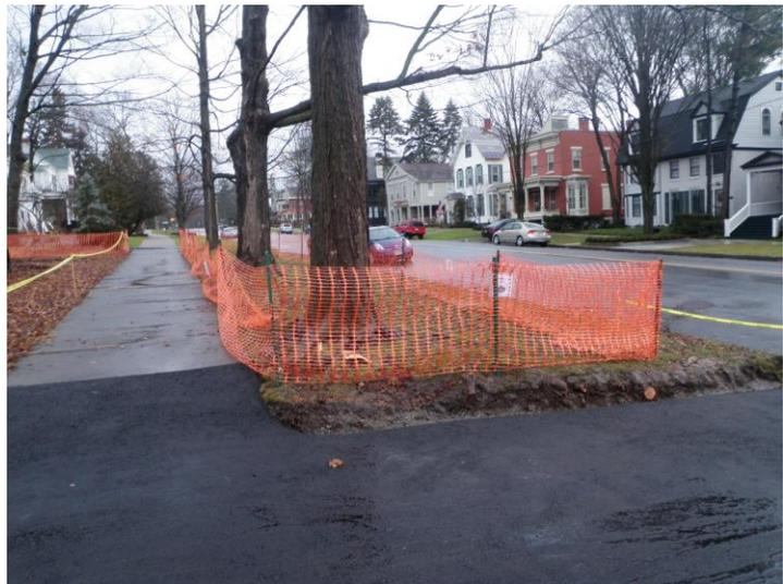
**Image 3:** This is an example of tree protection at a construction site. While the trees are protected and the disturbed roots were not torn, but cleanly cut; it could be argued that all disturbance to these trees could have been avoided if the site was accessed from the rear alley only.
