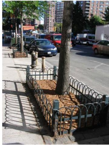
**Image 16:** Shows a comparison of how some sidewalk tree pits in Saratoga Springs are constructed, versus an example of how a tree pit is ideally constructed. The larger protected tree pit offers more rooting volume, access to moisture and oxygen for the tree, which will likely cause less damage to the sidewalk.
